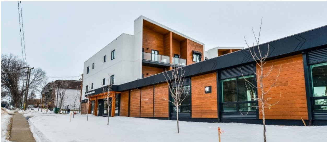
Figure 20. Street frontage showing the housing to the left and amenity wing to the right, Jason Surkan.
